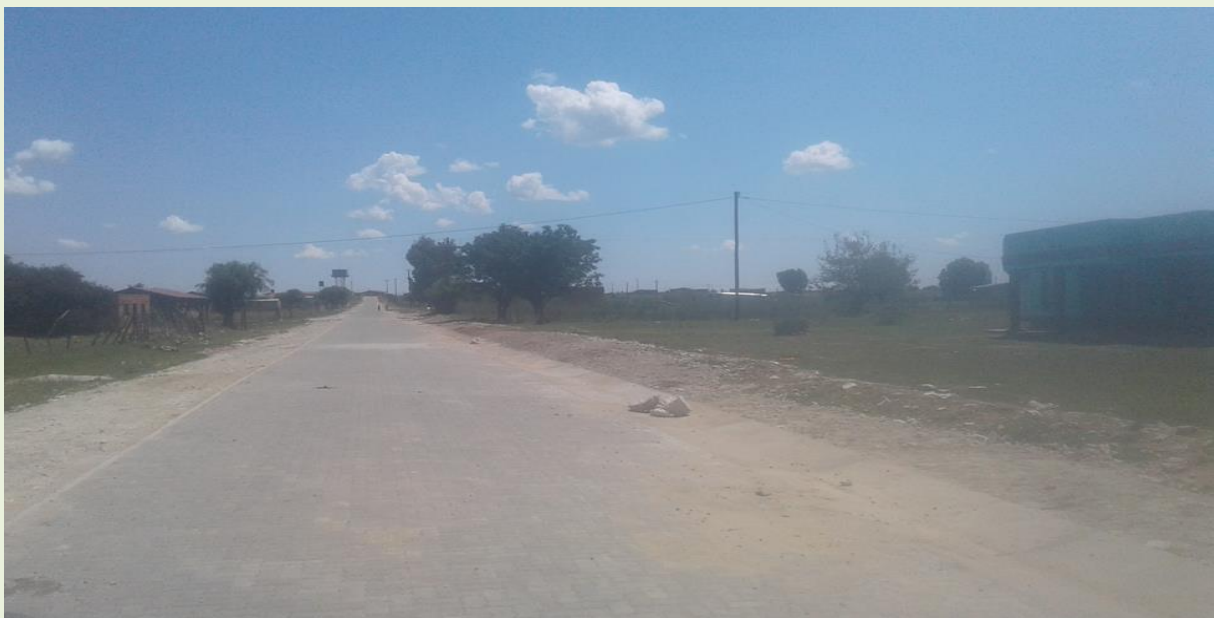
Kokomeng village Access Road completed in 2020/2021 . The roads was satisfactorily completed
