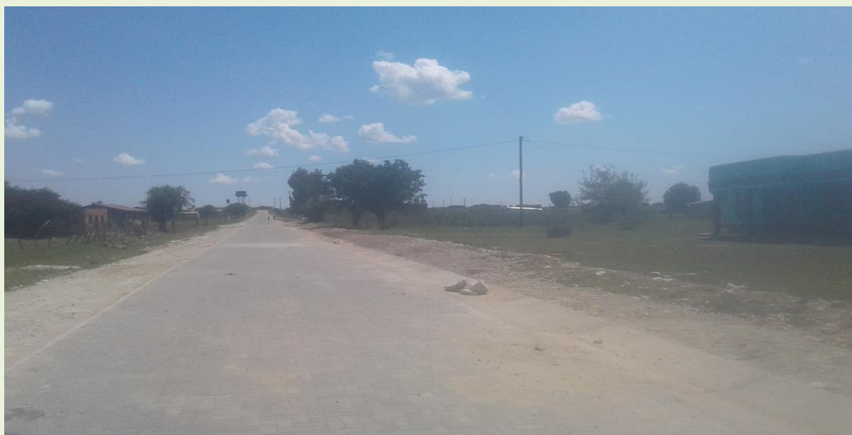
Kokomeng village Access Road completed in 2018/19
