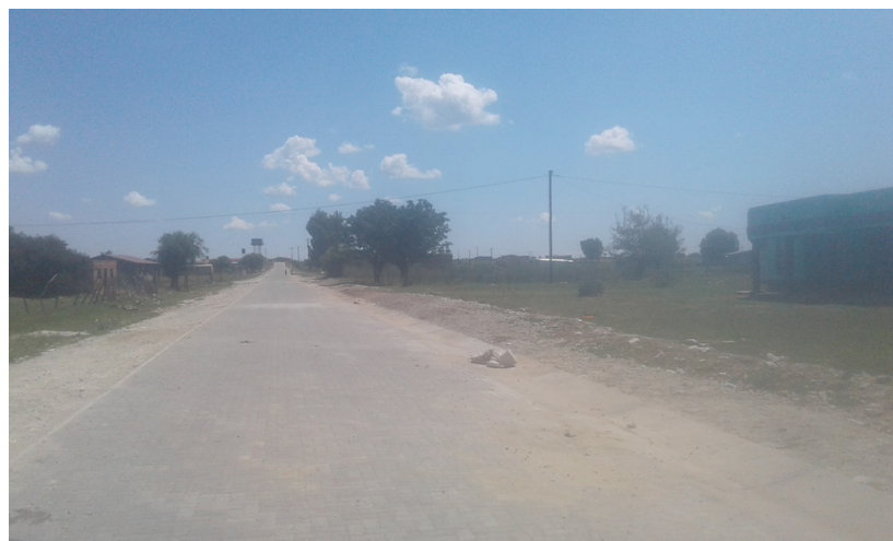
Kokomeng village Access Road completed in 2017/18
