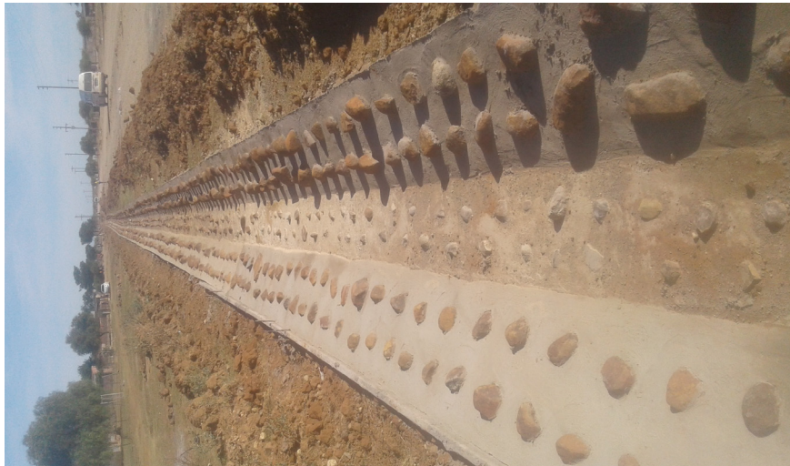
Matsheng village Stormwater channel completed in 2016/17
