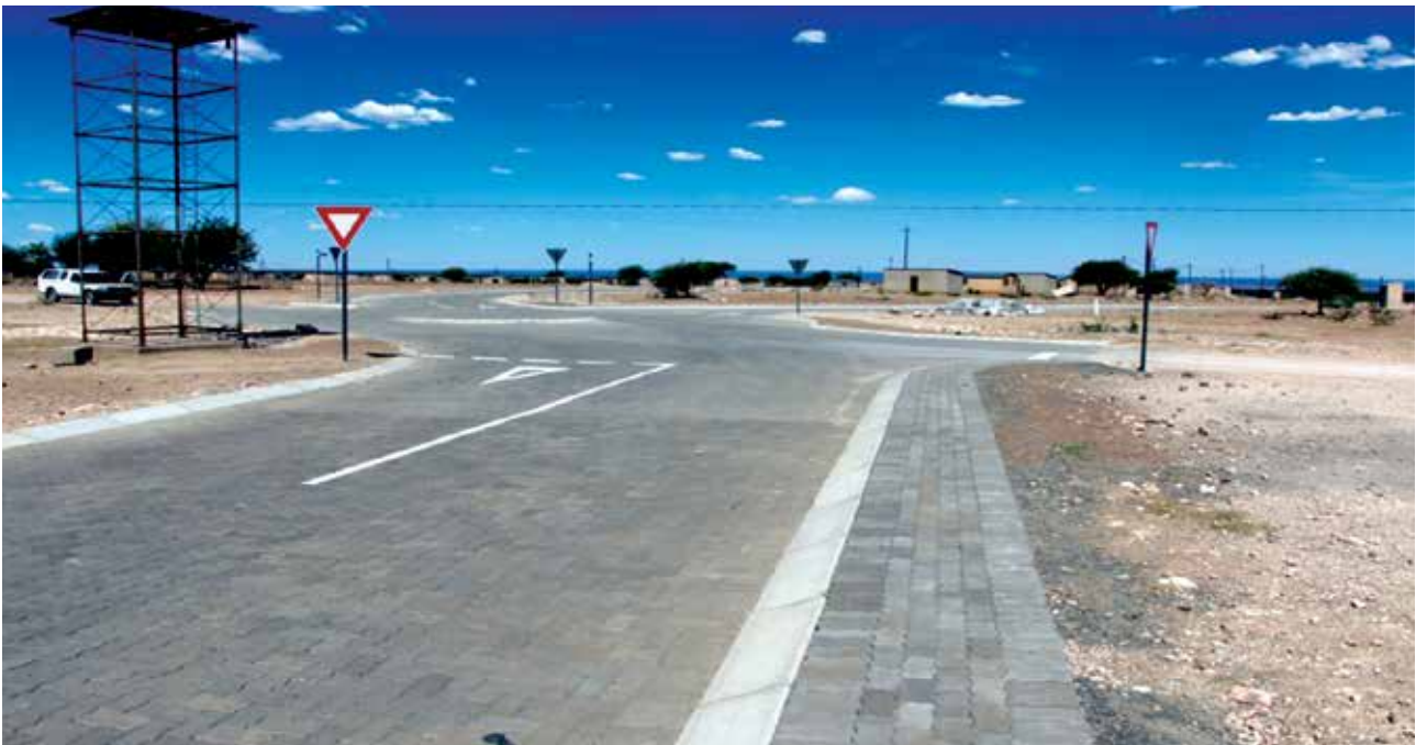
Rietfontein village Access Road Completed in 2015/16
